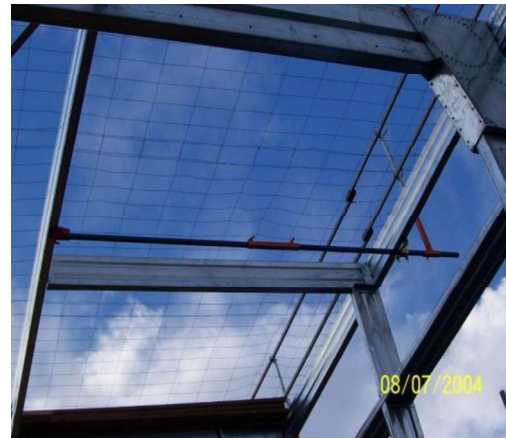
Figure 15: An example of safety mesh installed prior to roof construction.
